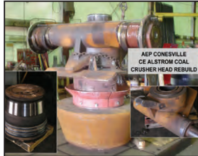
Coal Crusher Rebuild
